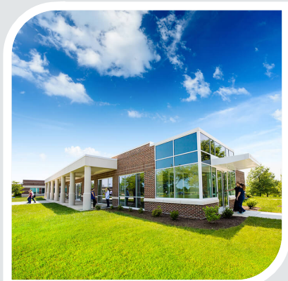
Winchester Campus 1775 North Sector Court Winchester, VA 22601
